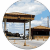
Canopies and Prefab Buildings
